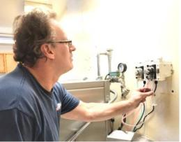
The dishwasher system has been upgraded to use liquid detergent and rinse agent getting rid of the old bulky system that wasn't working properly. The new system has special pumps that
